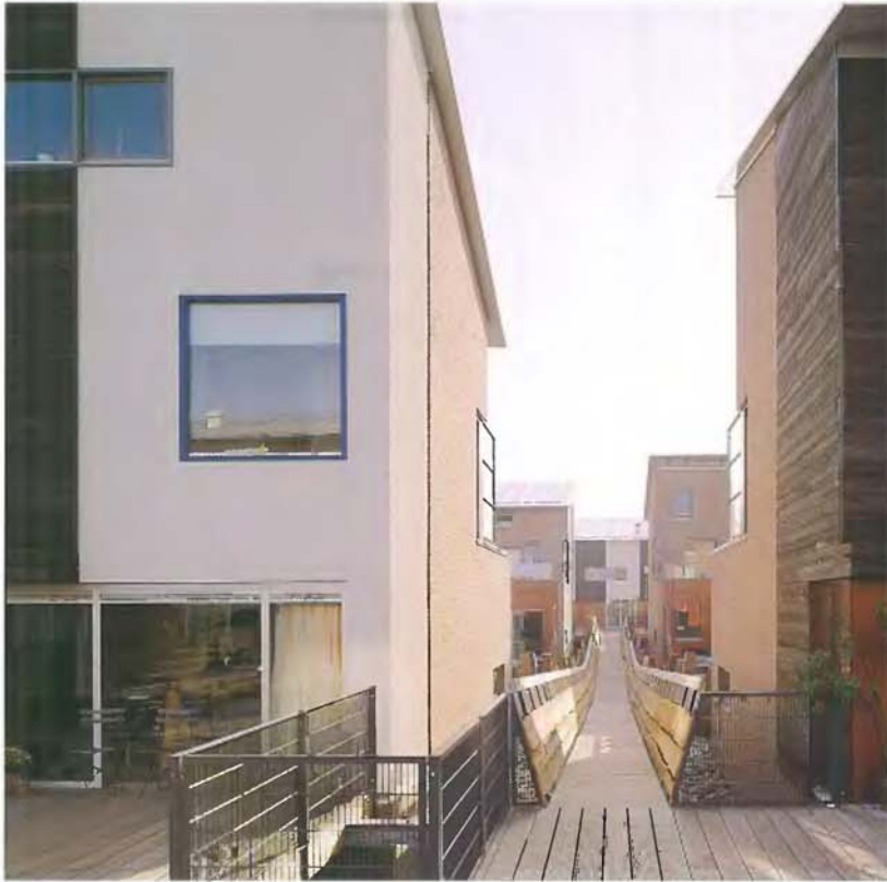
A bridge connects the various islands. The gaps between the wooden planks of the platform, built in the traditional scaffolding manner, let filtered light through to the interior.
