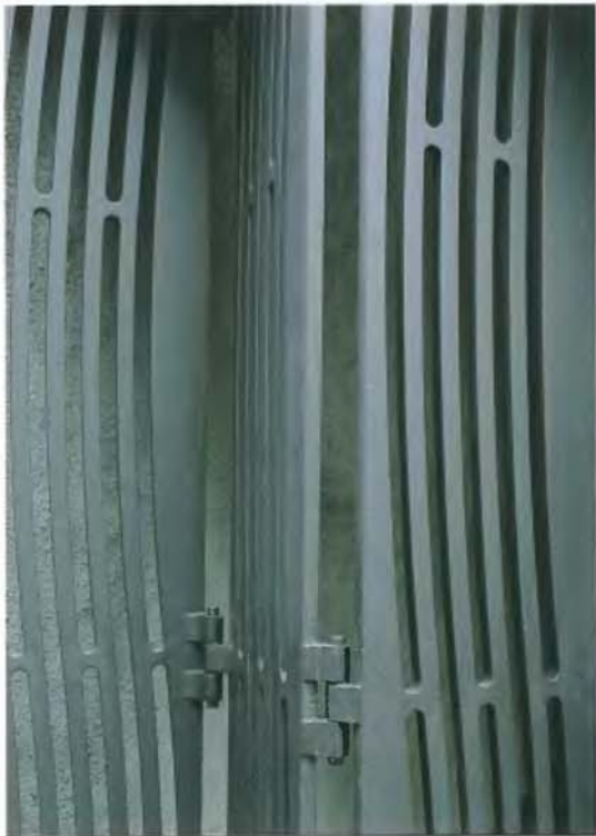
Front view of the main facade, characterised by the unusual cast iron curtain, which as it sways endows the whole scene with fluidity and dynamism. The detail below shows how the individual links of the curtain are joined together.
