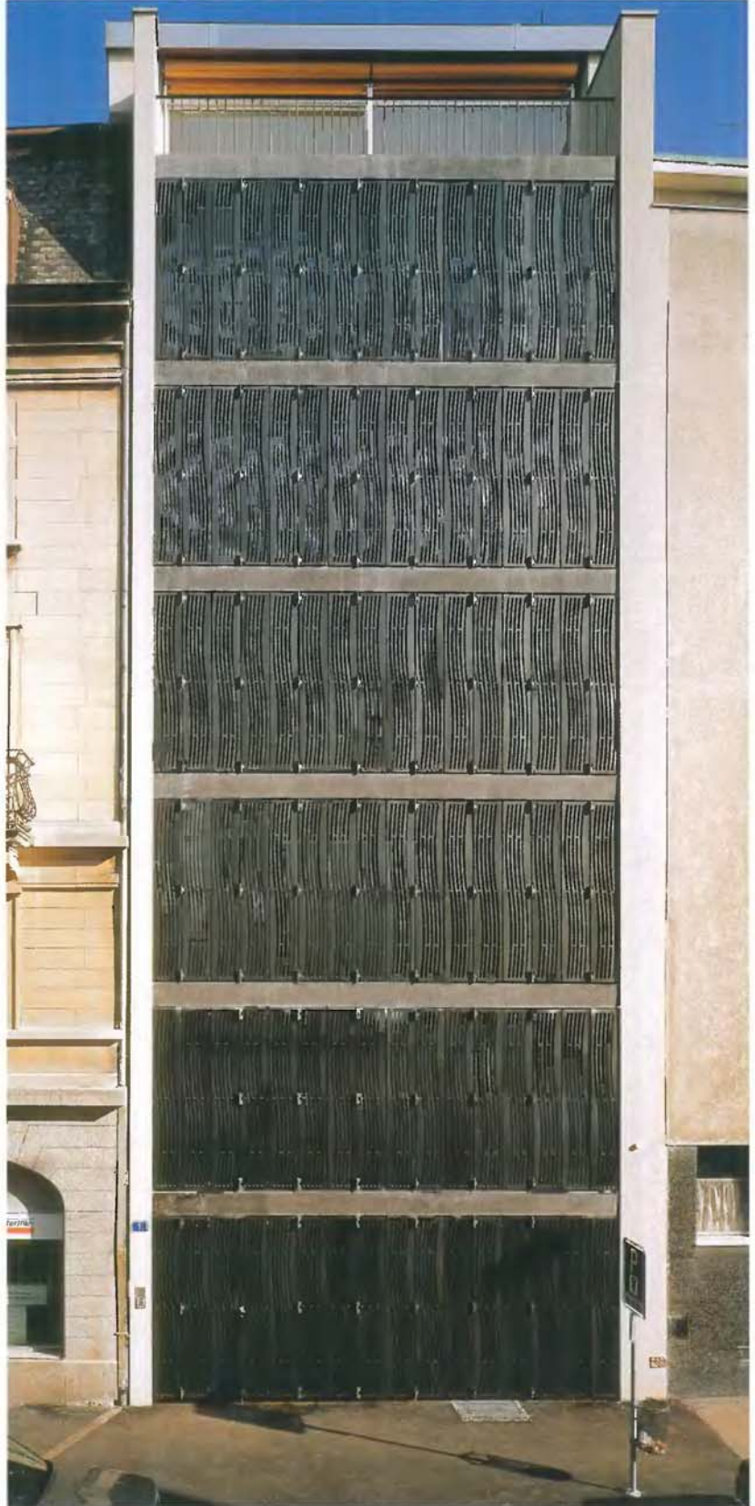
Front view of the main facade, characterised by the unusual cast iron curtain, which as it sways endows the whole scene with fluidity and dynamism. The detail below shows how the individual links of the curtain are joined together.
