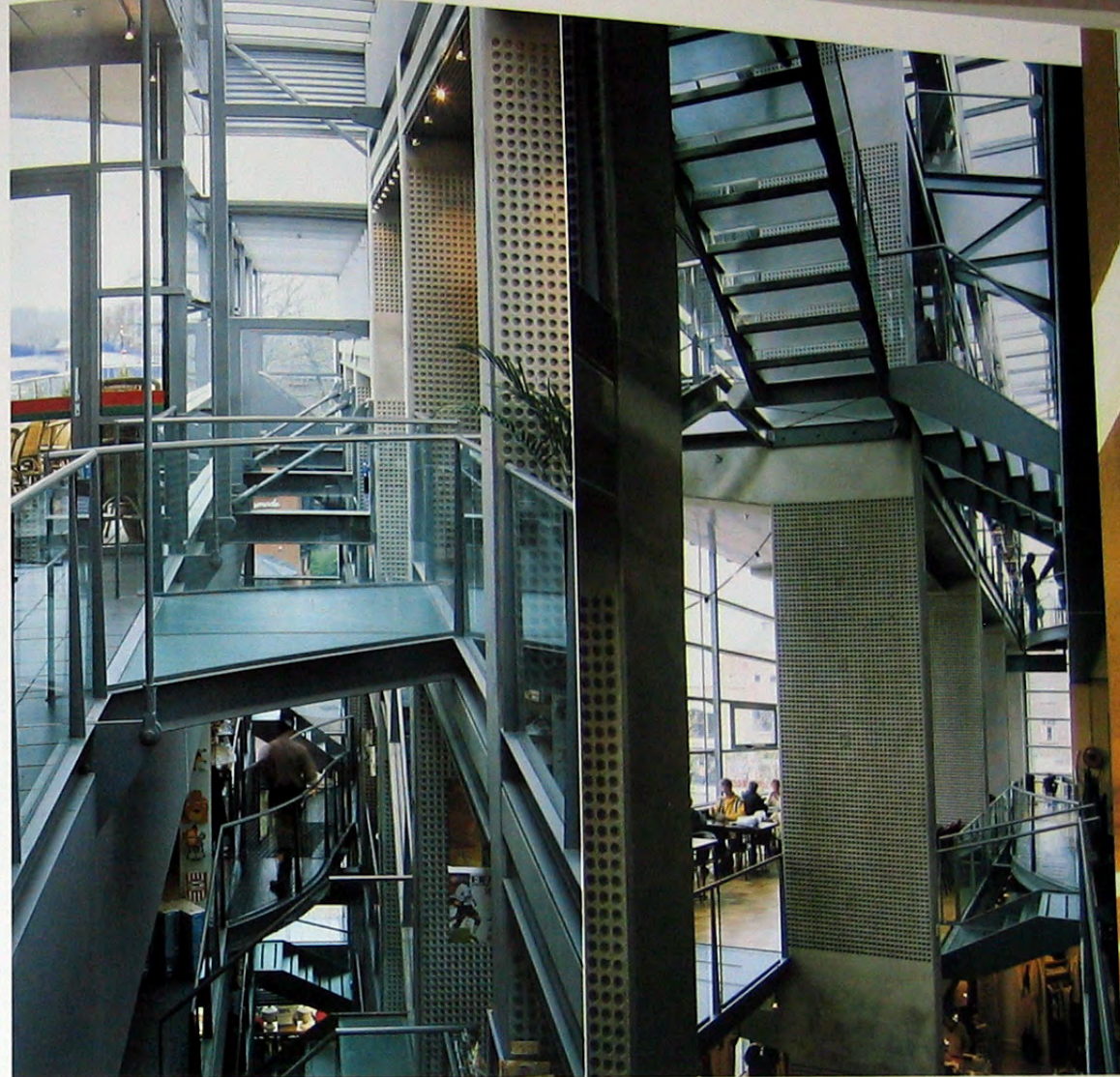
above left and above: 'Gangplanks' link the existing building to the annexe, crossing a 1.5-metre-deep atrium which rises the full height of the building.
