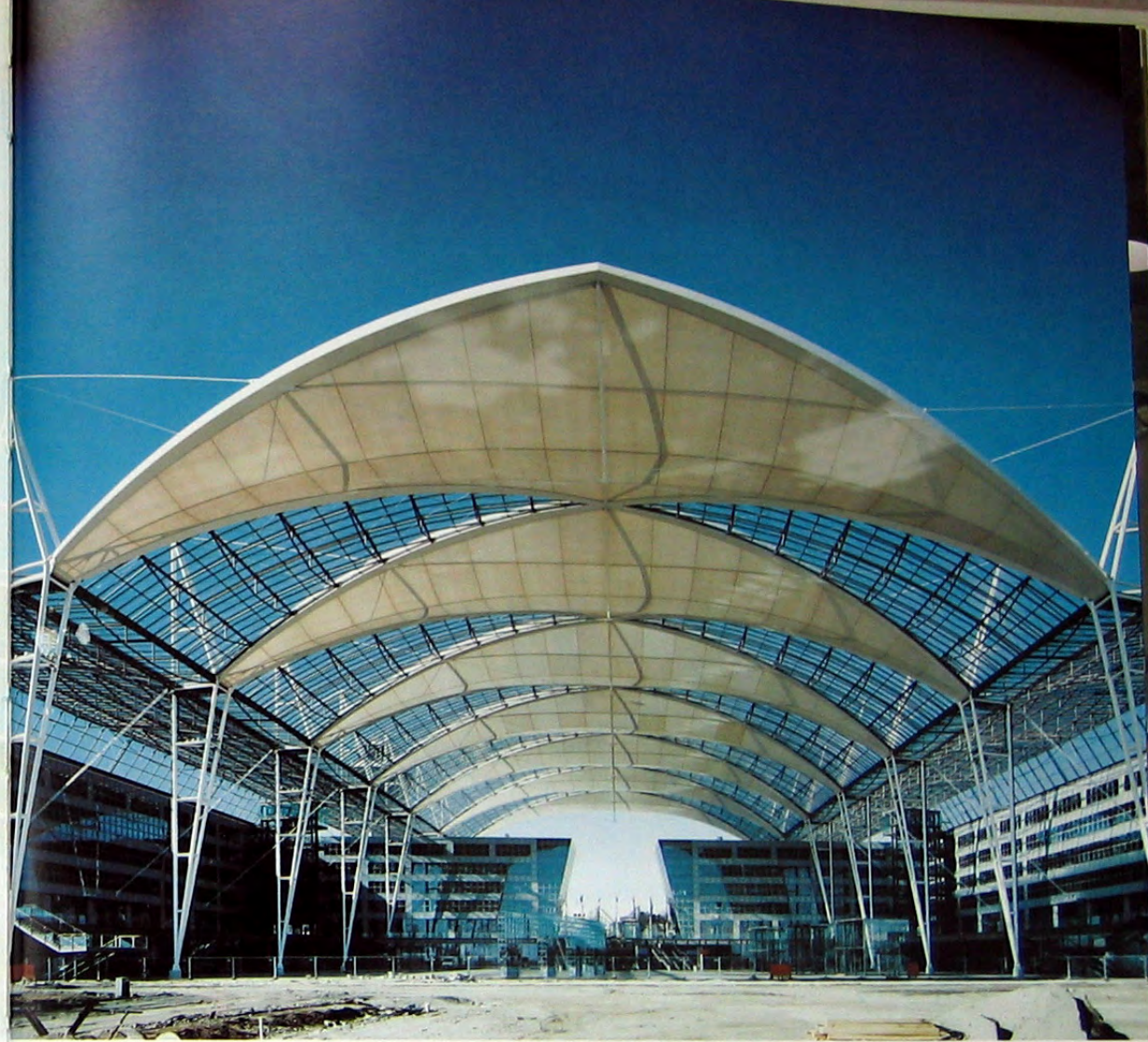
Between the masts the main steel beams run diagonally. The glazed sections between the diamond-shaped membranes consist of clear laminated glass with a substructure of steel pipe, trusses and tension rods.
