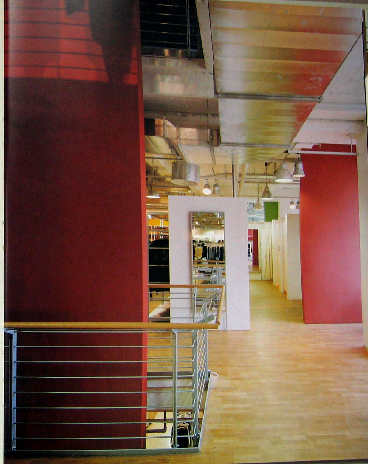
opposite: The bulk of the sales floor partition walls were removed and those that stayed were painted white or rust-red; false ceilings were also stripped away to leave pipework visible – intriguing new vistas were opened up in the process.
