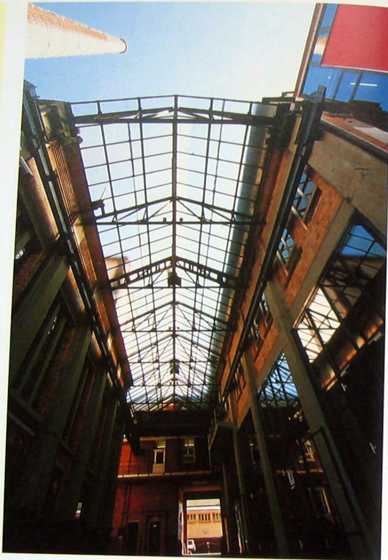
above: The firm of Friedrich Dick decided to get involved in the rejuvenation of its former massive industrial premises; the new commercial initiative did not abandon the structural relics of the past, such as the original roof girders.
