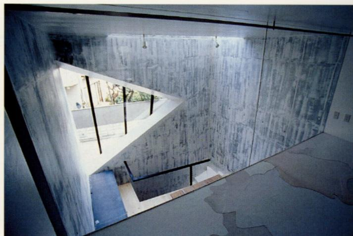
The walls are clad in high and wide expanses of exposed concrete. The floors are done almost entirely in unstained wood, the only exception being the unique flooring material used in the mezzanine: leather.
