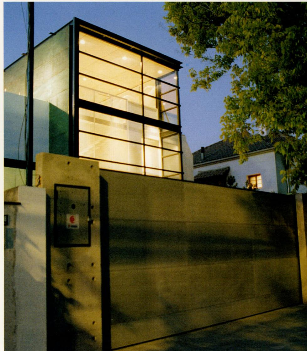
A metal structure was used to create a vertical plane that crosses the house lengthwise, forming the access toward the street. This plane folds to form the ceiling, and the three remaining sides are glazed. The exterior wall is clad in copper, which was given a green patina.
