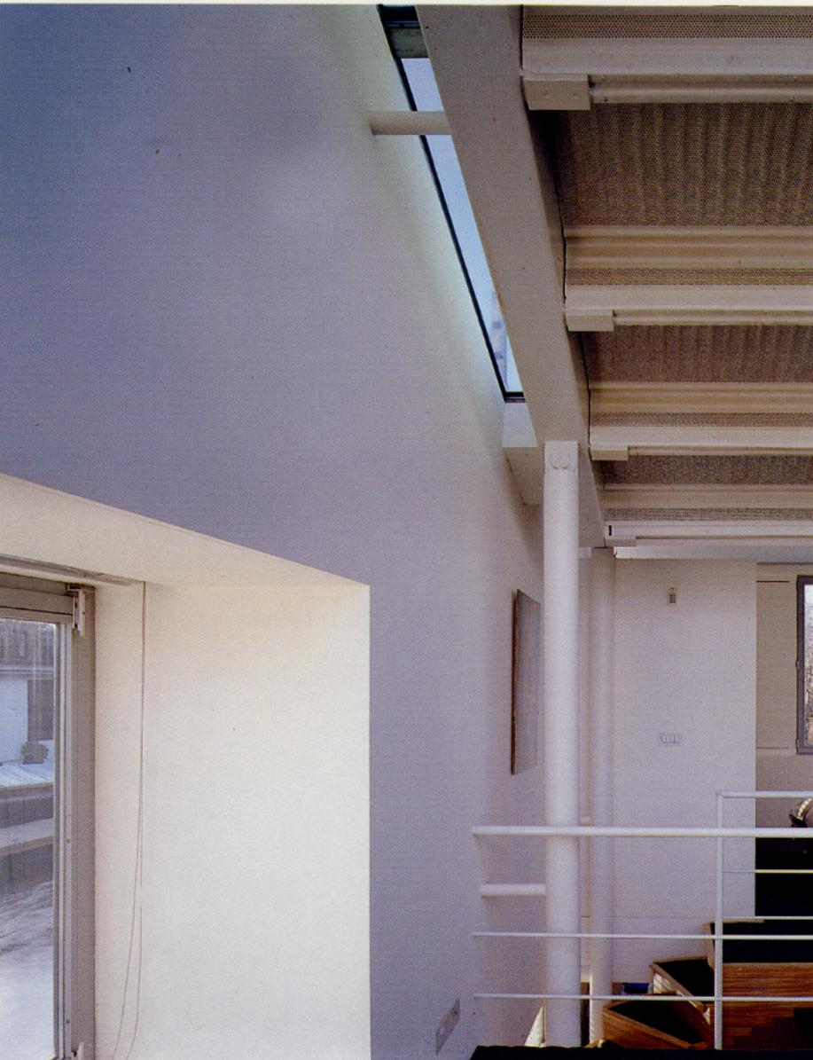
A metal valley-roof supported on perforated metal troughs and a steel frame is carried on two pairs of steel columns. This structure is dissociated from the perimeter walls and independent of the galleries and volumes below.
