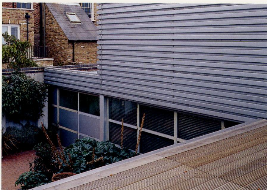
The design of the workshop section was governed by the need to maintain the two-story enclosure of the adjacent buildings and to keep the level of the roof below the single-story wall of the gardens on the north. The roof and all of the wall planes are dissociated by glazing.
