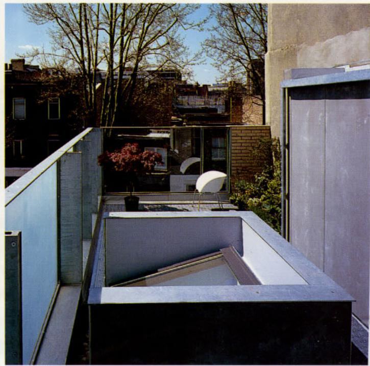
The superstructure is simple, consisting of planes of well insulated cavity masonry walls with wood and steel floor plates. This sturdy construction is combined with a relatively sophisticated services installation consisting of a condensing boiler, which provides under-floor heating with heat reclaim ducted ventilation to the bedrooms and bathrooms.
